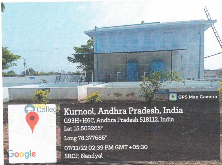
Sewage water treatment Plant
