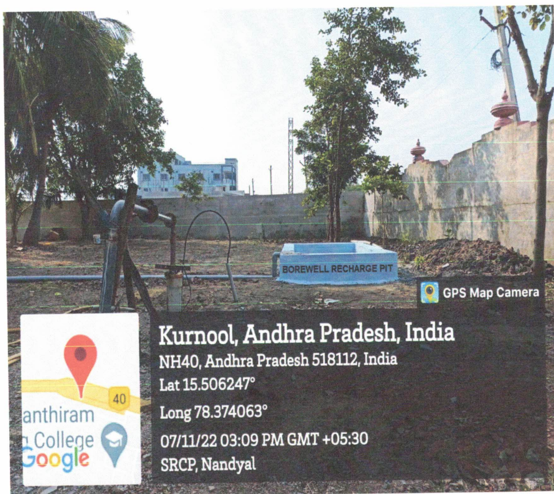
Borewell Recharge Pit
